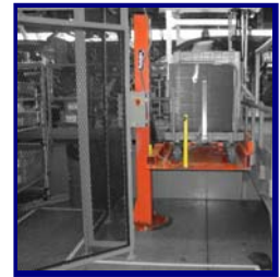
Example of Fencing
